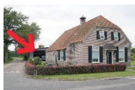
Trentsedijk 20 In open loods
